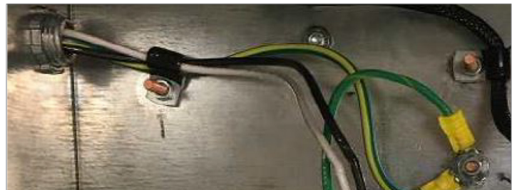
Connect PE from junction box to the welded stud in the power supply box.
