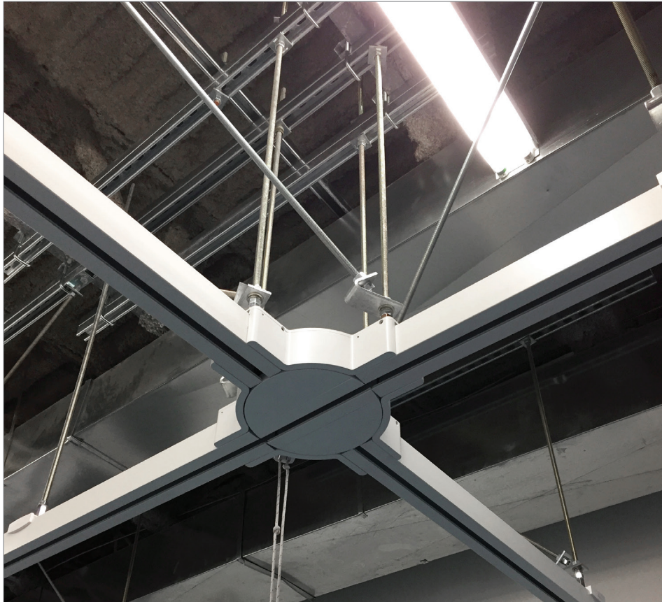
Typical turntable installation with Unistrut hardware and ½" (12.7mm) threaded rods.
