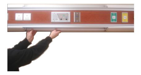
Replace the lens covers using the provided screws.
